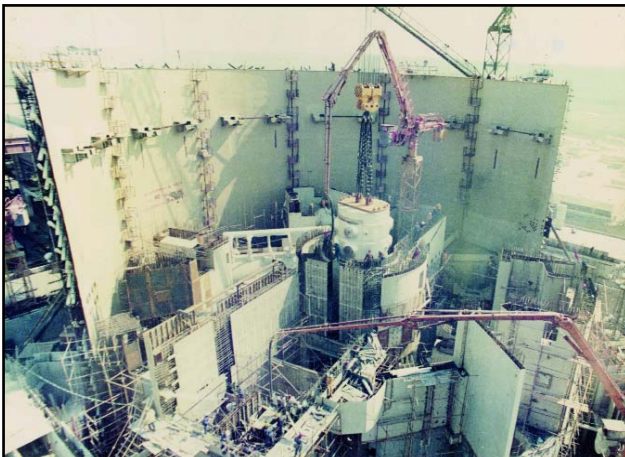
Mounting the reactor vessel, April 11, 1985
